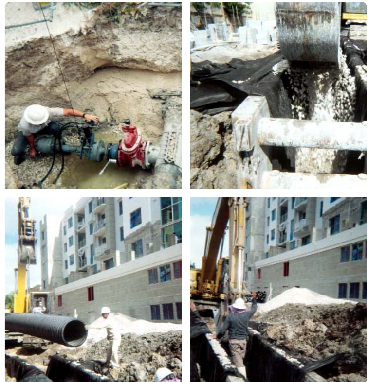
Underground Utilities Improvements
