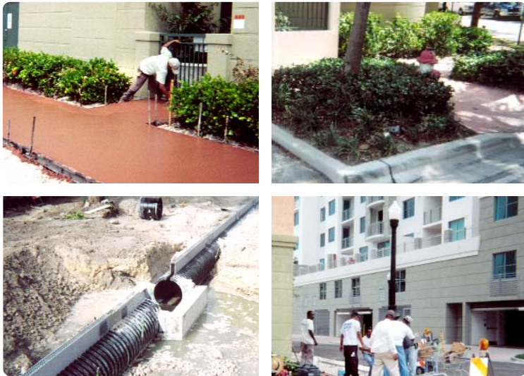
Street Improvements in Progress
