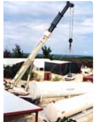
Utilities During Installation
