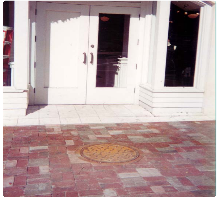
Street Level Drainage
