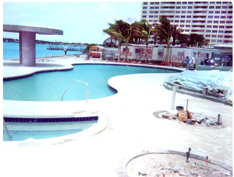
Pool and Deck Area Under Construction
