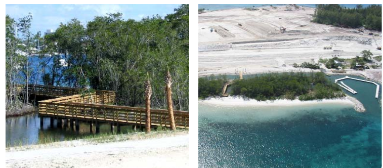
Recreational Features Under Construction
