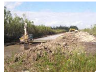
Levee and Site Construction Progress
