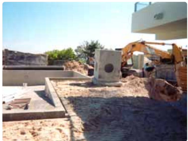
Pool Area Under Construction
