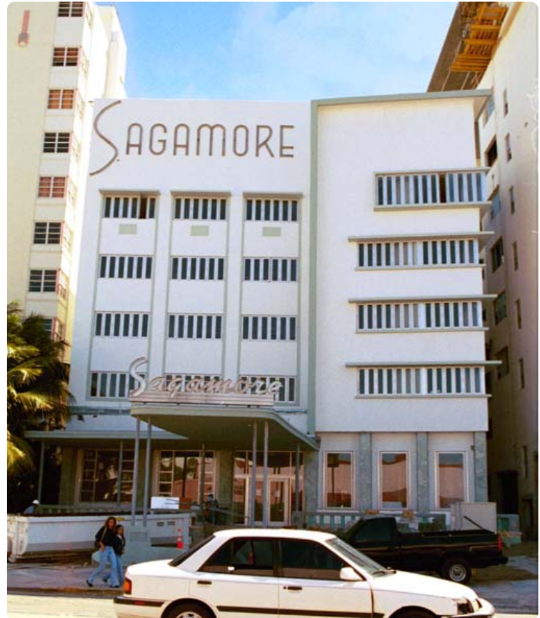
Collins Avenue View During Construction
