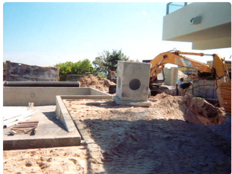
Pool Area Under Construction
