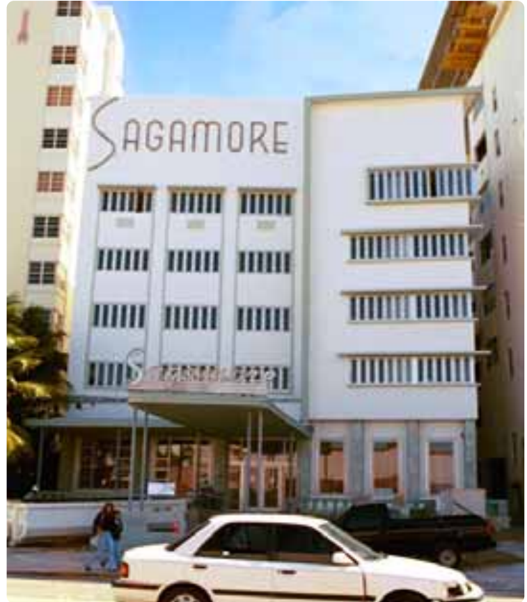
Collins Avenue View During Construction
