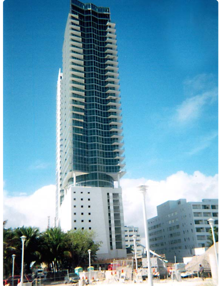
Resort Under Construction
