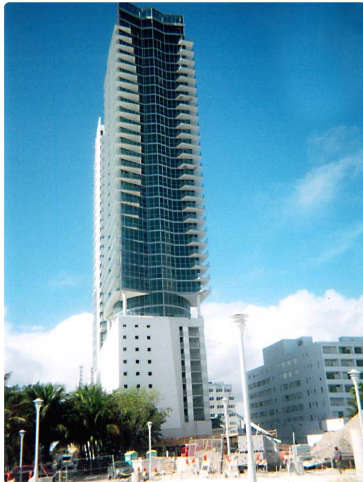
Resort Under Construction
