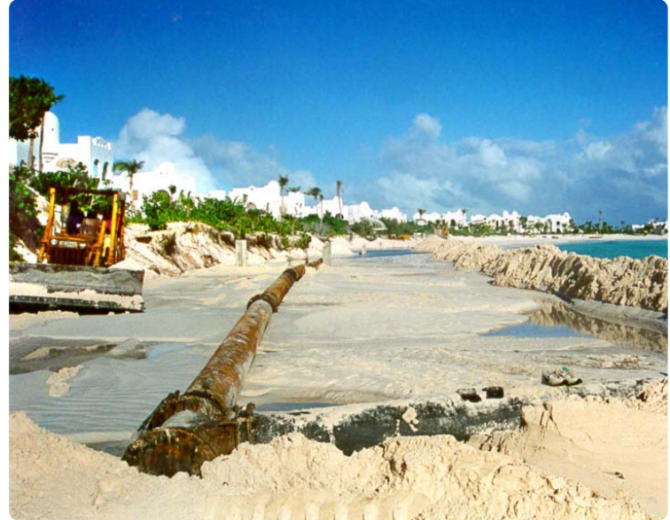
Earthworks & Dredging In Progress
