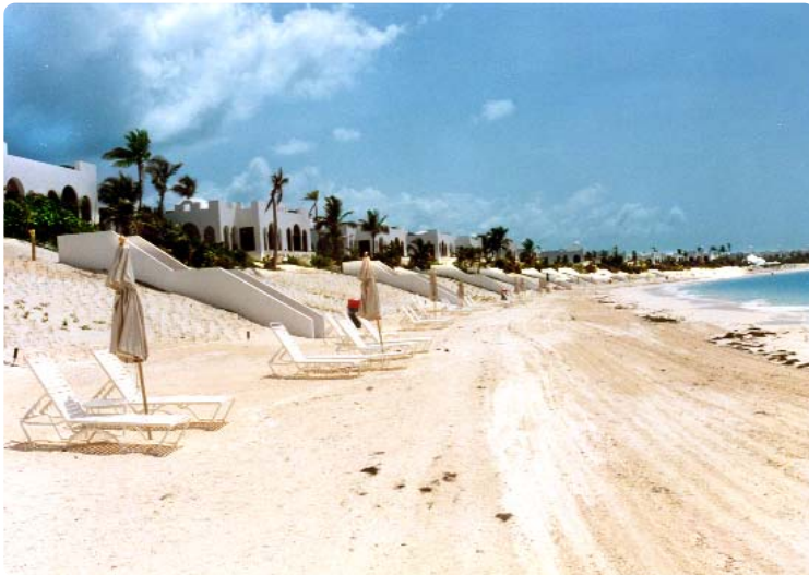
View of Beach Post Nourishment
