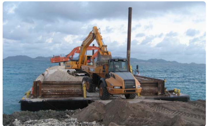
Earthworks in Progress for Beach Nourishment
