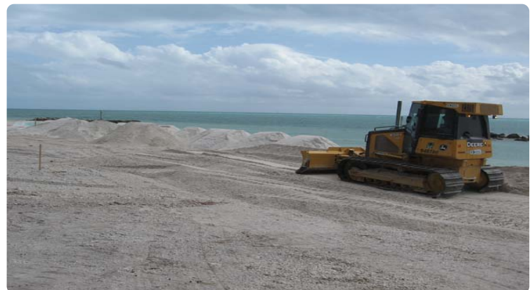
2007 Truck-Haul in Progress
