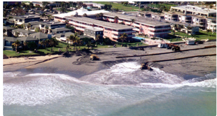
Beach Fill Under Construction
