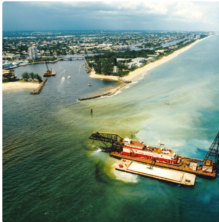
Dredging in Progress
