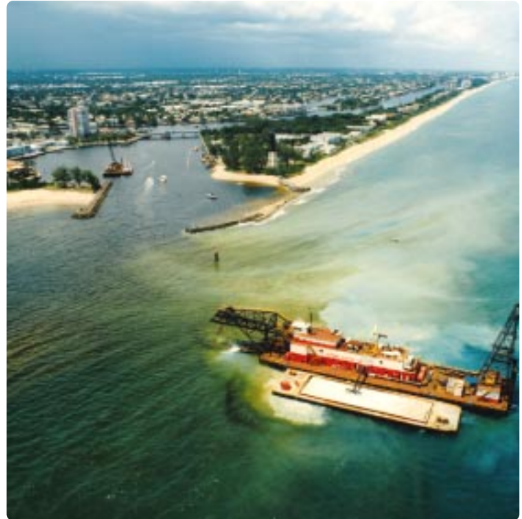
Dredging in Progress
