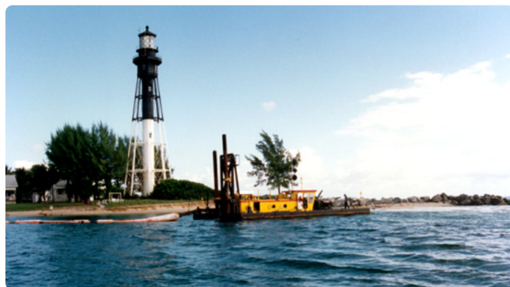
Within the Inlet Sand Dredging
