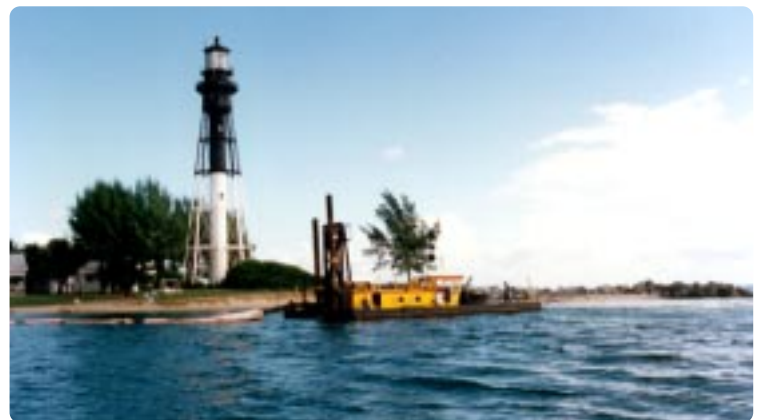
Within the Inlet Sand Dredging
