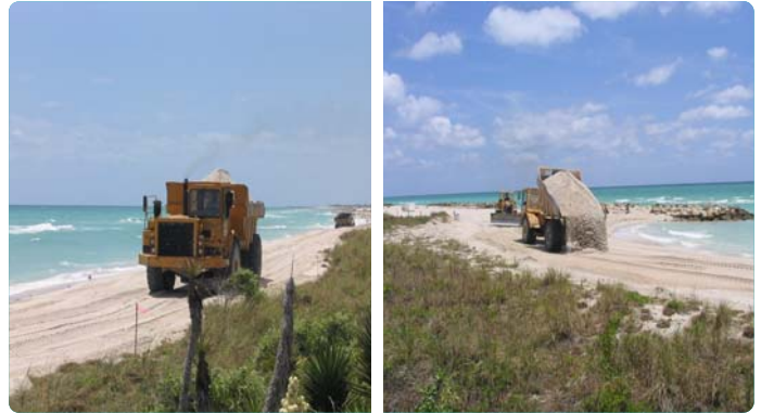
Truck Haul Sand Placement
