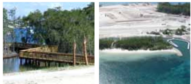
Recreational Features Under Construction
