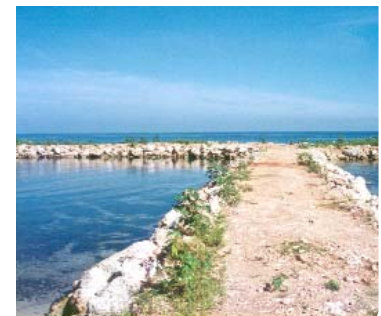
Construction of Coastal Structures
