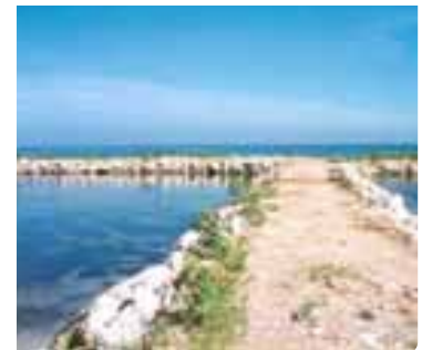
Construction of Coastal Structures
