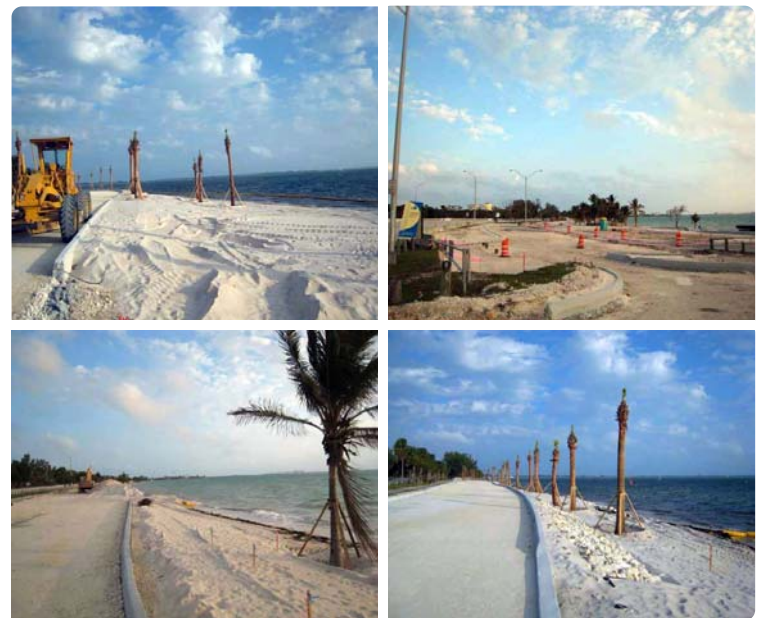
Shoreline and Stormwater Management Construction
