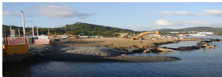
Land Reclamation Under Construction
