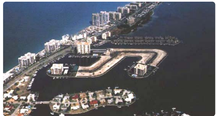
Beach Nourishment in Progress
