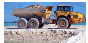
Construction of Entrance Channel
