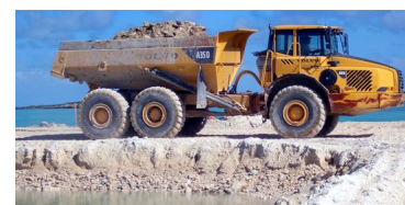
Construction of Entrance Channel
