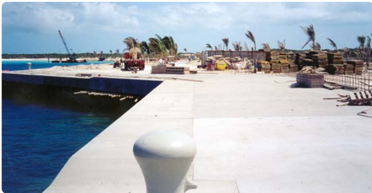
Enlarged Concrete Pile Cap
