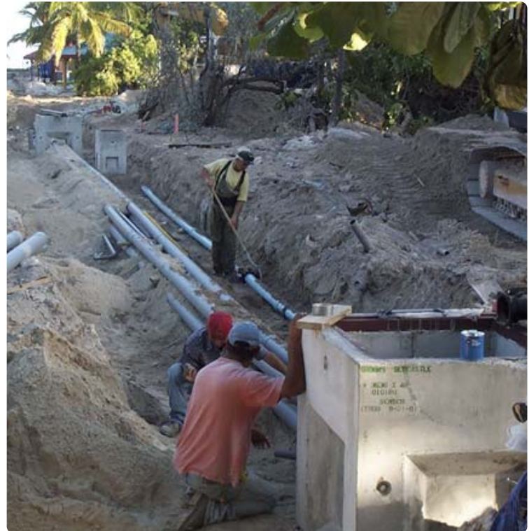
Underground Utilities Installation
