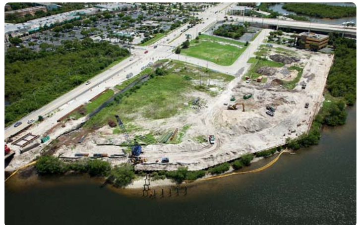
Aerial View of Construction
