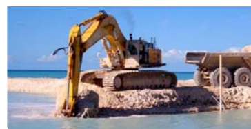
Construction of Entrance Channel in Progress
