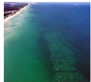
Reef Construction in Progress
