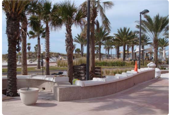
Close up View of Wave Dissipating Wall
