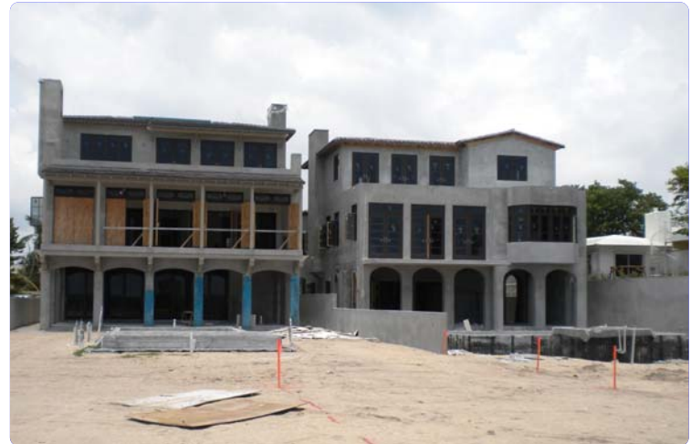
Residences Under Construction
