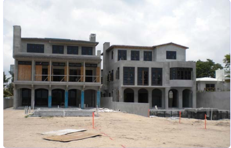
Residences Under Construction
