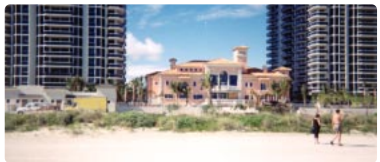
Auxiliary Structures & Pool Area
