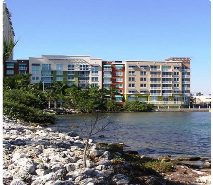
View of Cité with Revetment and Seawall
