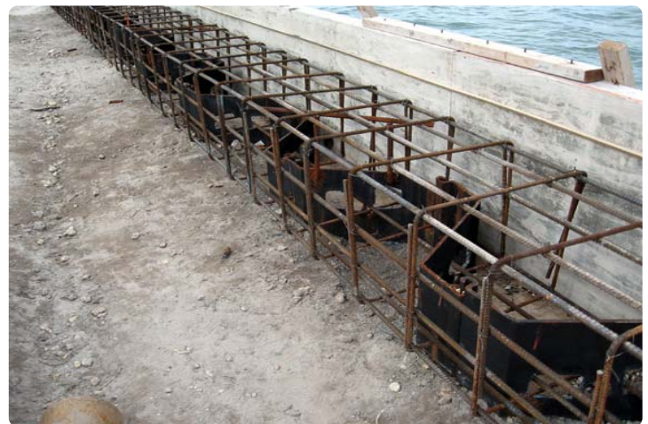
Reinforcement for New Cap
