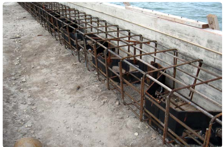
Reinforcement for New Cap
