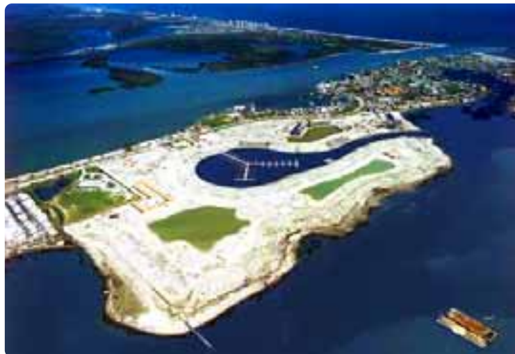
Pre-construction Harbour Isle
