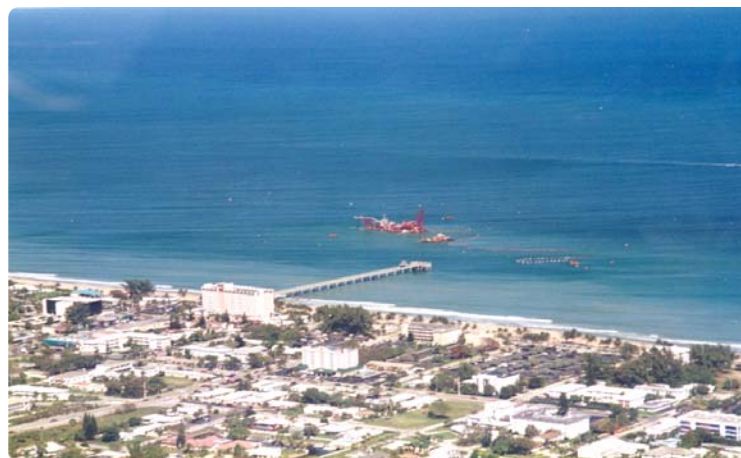
Dredge Excavating Sand from Borrow Area 1 during the 1998 Renourishment Project
