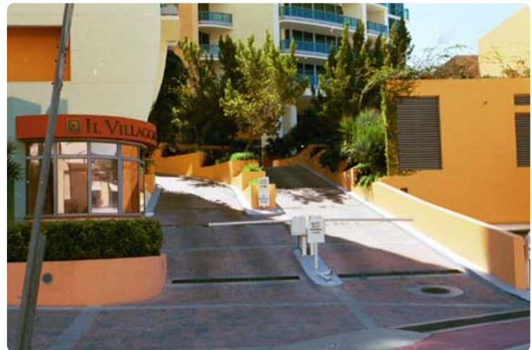
Parking Garage showing Storm Drainage
