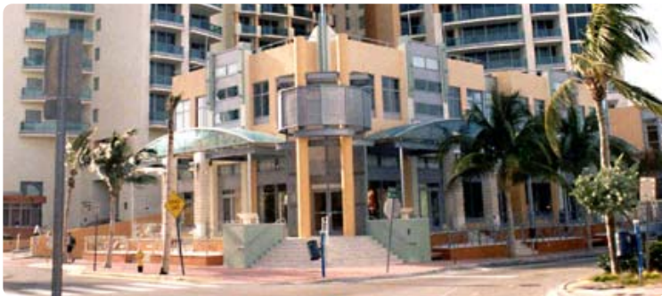
2-Story Retail Building
