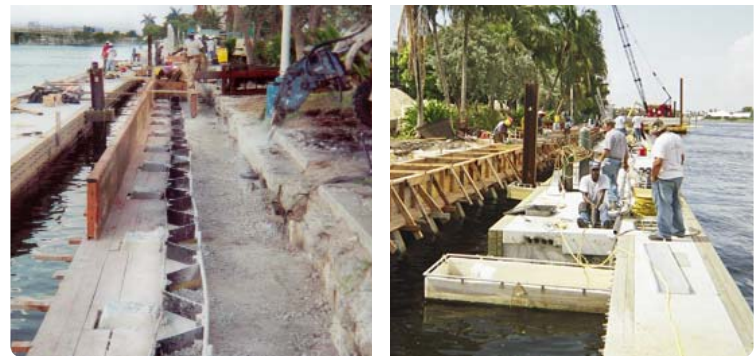
Bulkhead and Dredging Construction
