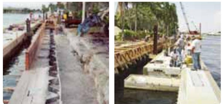
Bulkhead and Dredging Construction
