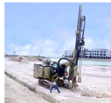
Construction in Progress
