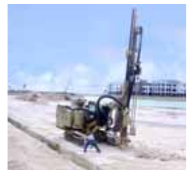
Construction in Progress
