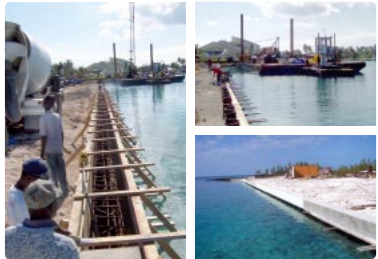
Marina Construction in Progress
