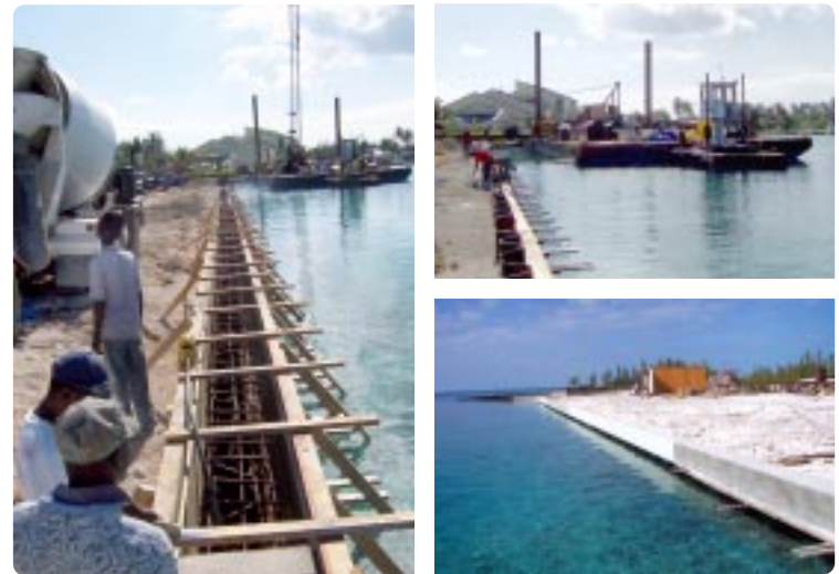
Marina Construction in Progress
