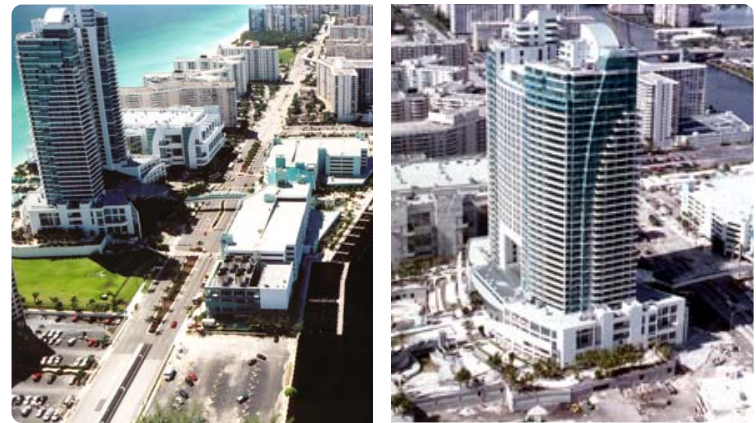
Building & Docking Facilities Under Construction
