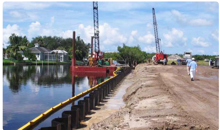
Bulkhead Under Construction
