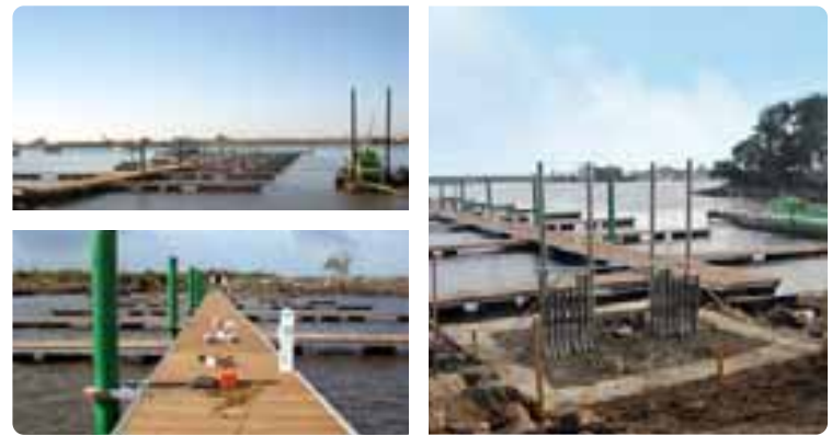
Marina Under Construction
