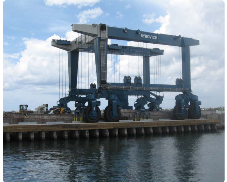
Marine Travelift Piers
