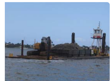
Floating Docks and Dredging
