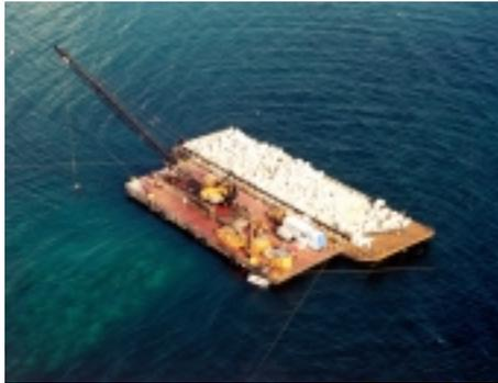
Steel cables are typically used for the winch lines of a barge mooring system. However, floating lines with equivalent strength of the steel cable were utilized by conventional deck winches. The floating lines minimized the risk of cable-dragging in close proximity to reef edges. In addition, all barge towing operations used floating lines exclusively.
