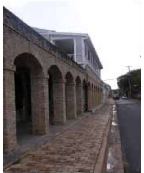
A newly paved sidewalk and new street improve the look of Frederiksted's main commercial thoroughfare, Strand1 Street.
