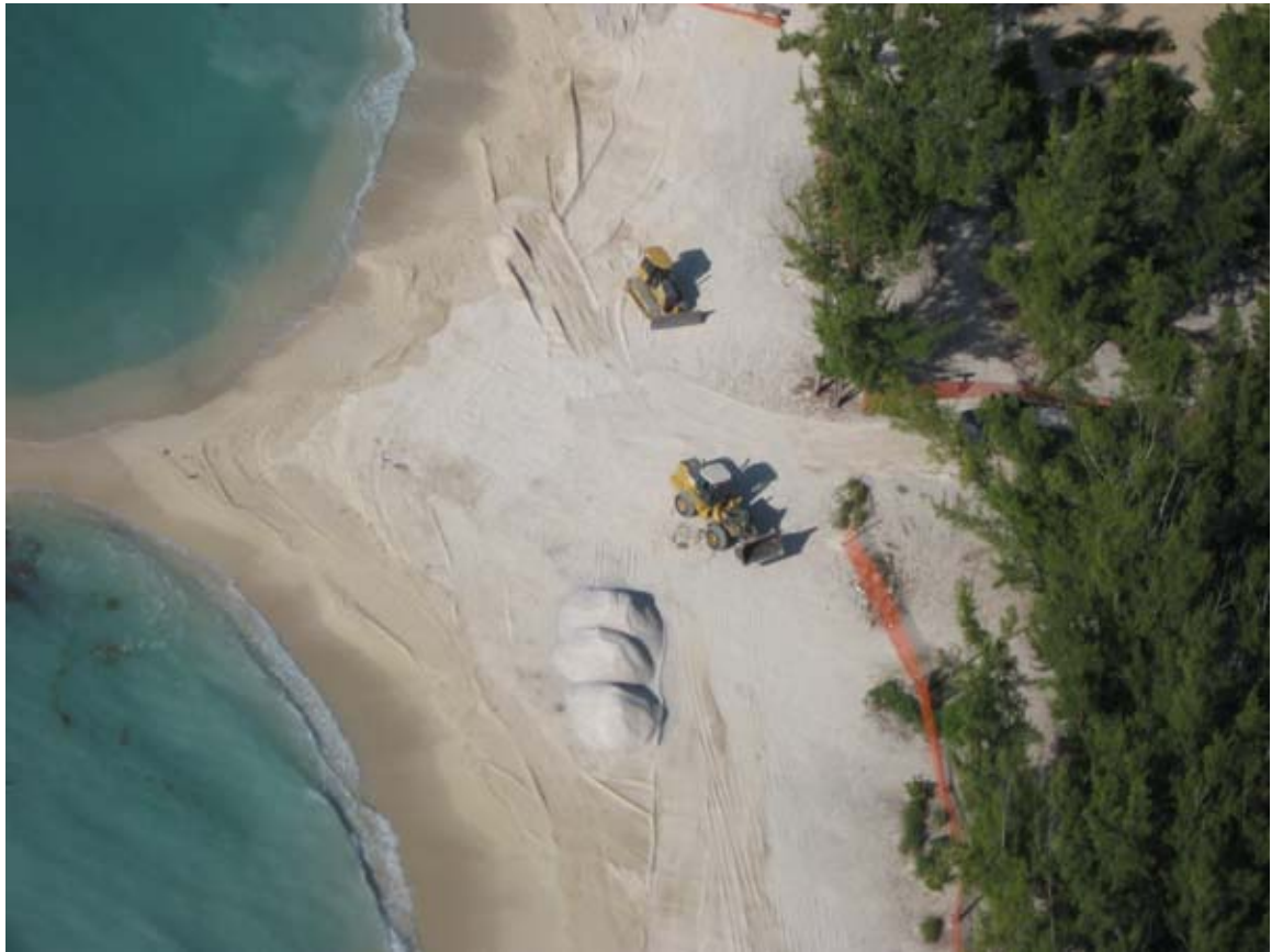
Aerial Photo during construction
