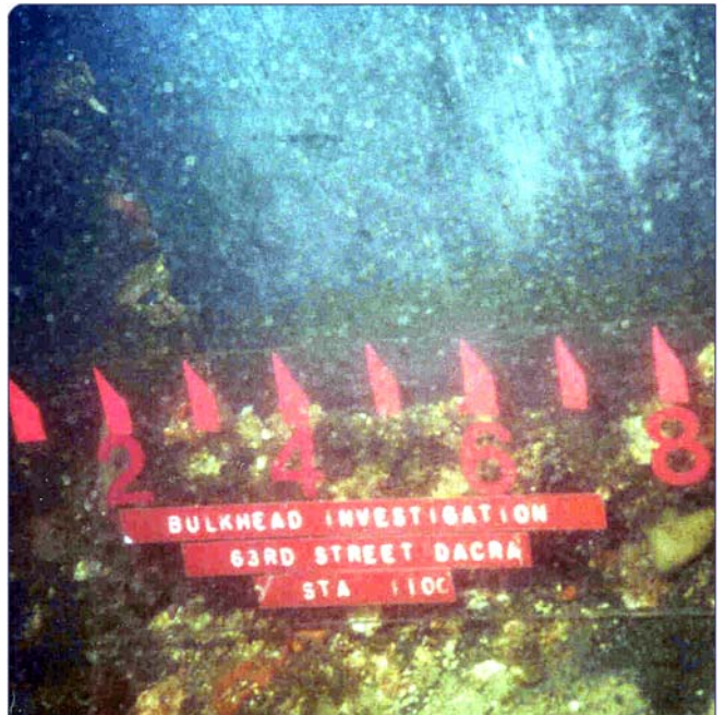
Underwater photograph of steel sheet piling
