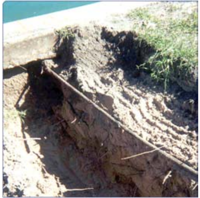
Exploratory excavation to evaluate condition of the tie backs.
