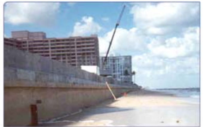
Typical oceanfront seawall
