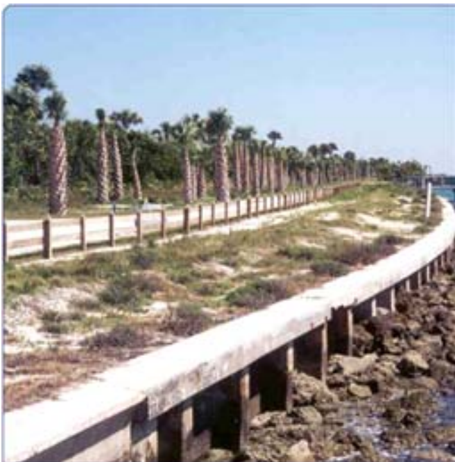
Typical coastal seawall
