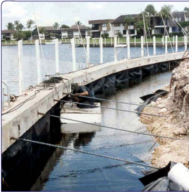
Typical bulkhead under construction
