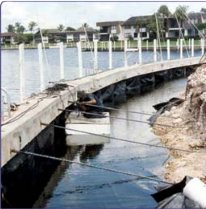
Typical bulkhead under construction
