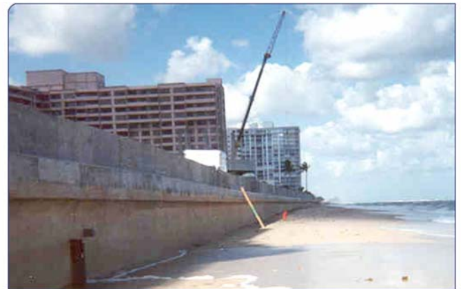
Typical oceanfront seawall
