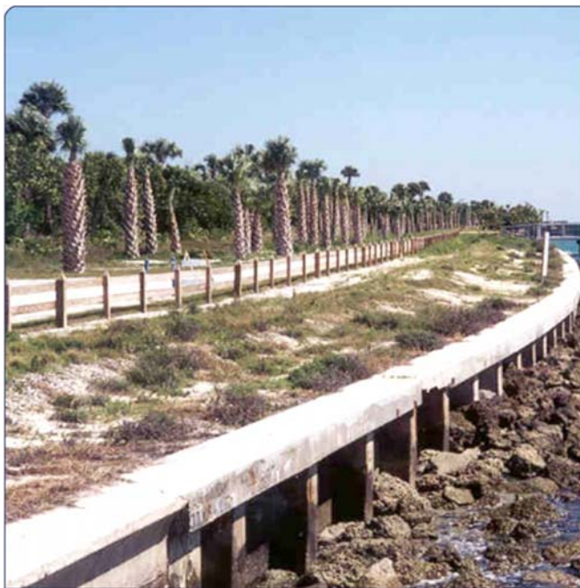
Typical coastal seawall
