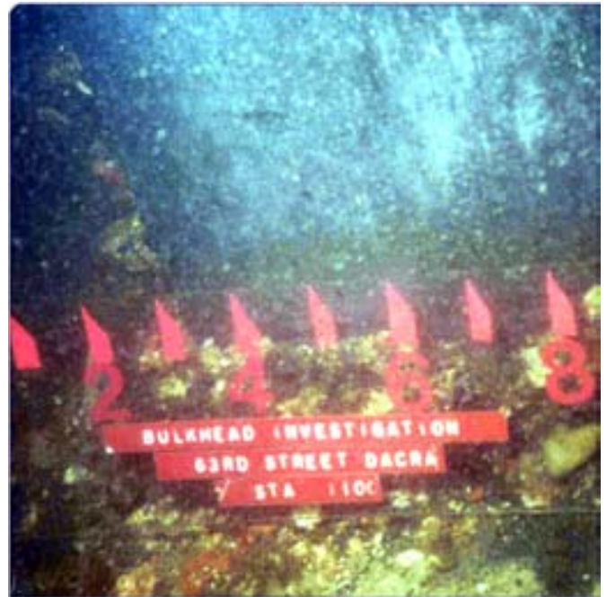
Underwater photograph of steel sheet piling
