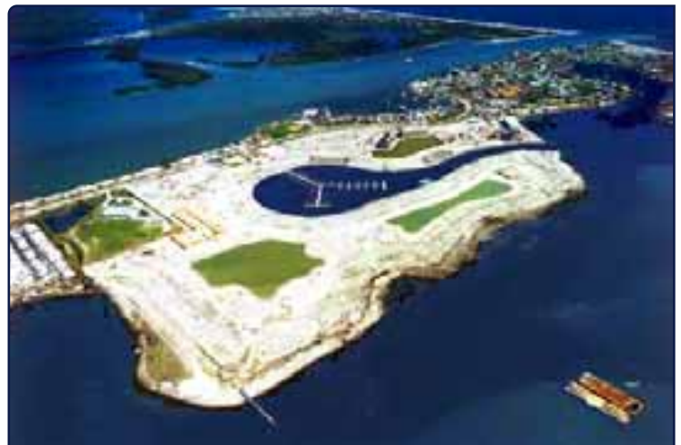
Figure 4: Pre-construction Harbour Isle
