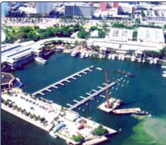
Miamarina: Miami, Florida (Under Construction)
